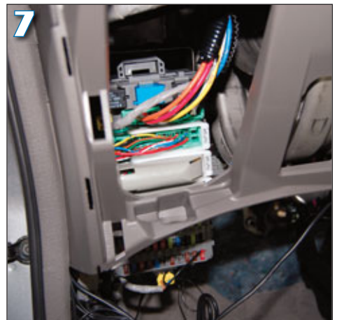
7 The ignition wires are located in a junction box directly above the fuse box in gray sheathing.
